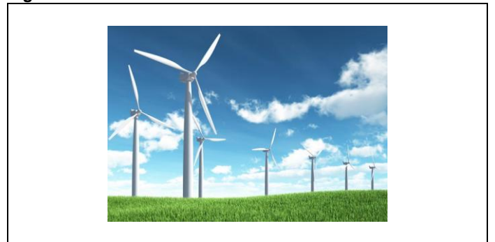
Figure 6. Wind Turbine Farm
